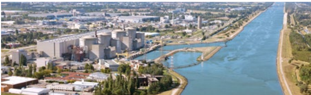
Tricastin Nuclear Power Plant (NPP)
